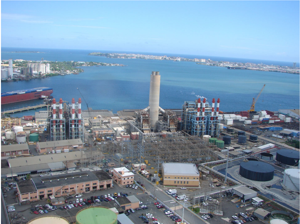
Figure 2-2 - San Juan Power Plant
