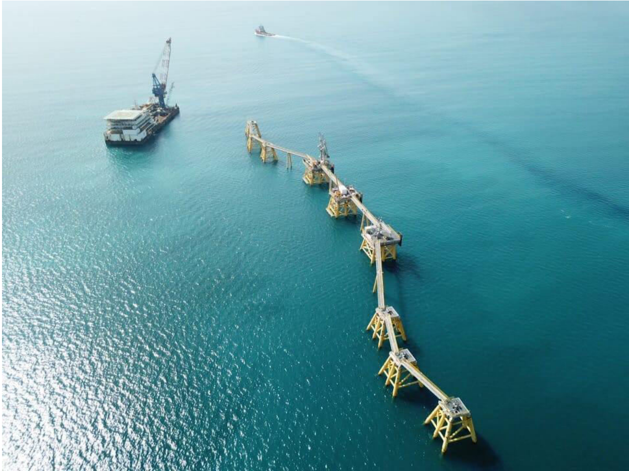
Figure 1-2: New Fortress Energy World-Scale, Old Harbour LNG Terminal
