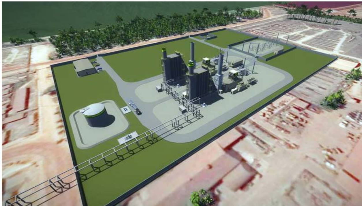
Figure 1-3: Jamalco Combined Heat and Power Plant
