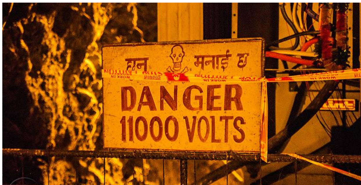
Adit tunnel, part of an unfinished Lanco Hydropower project. Teesta River – Sikkim, India
