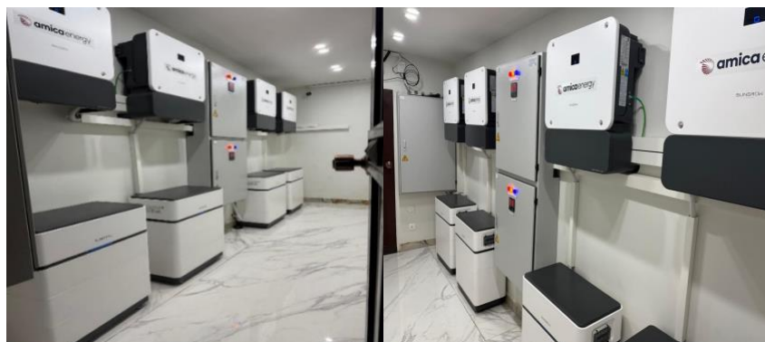
Figure 15: Gem Net 100kW/60kWh Hybrid System
