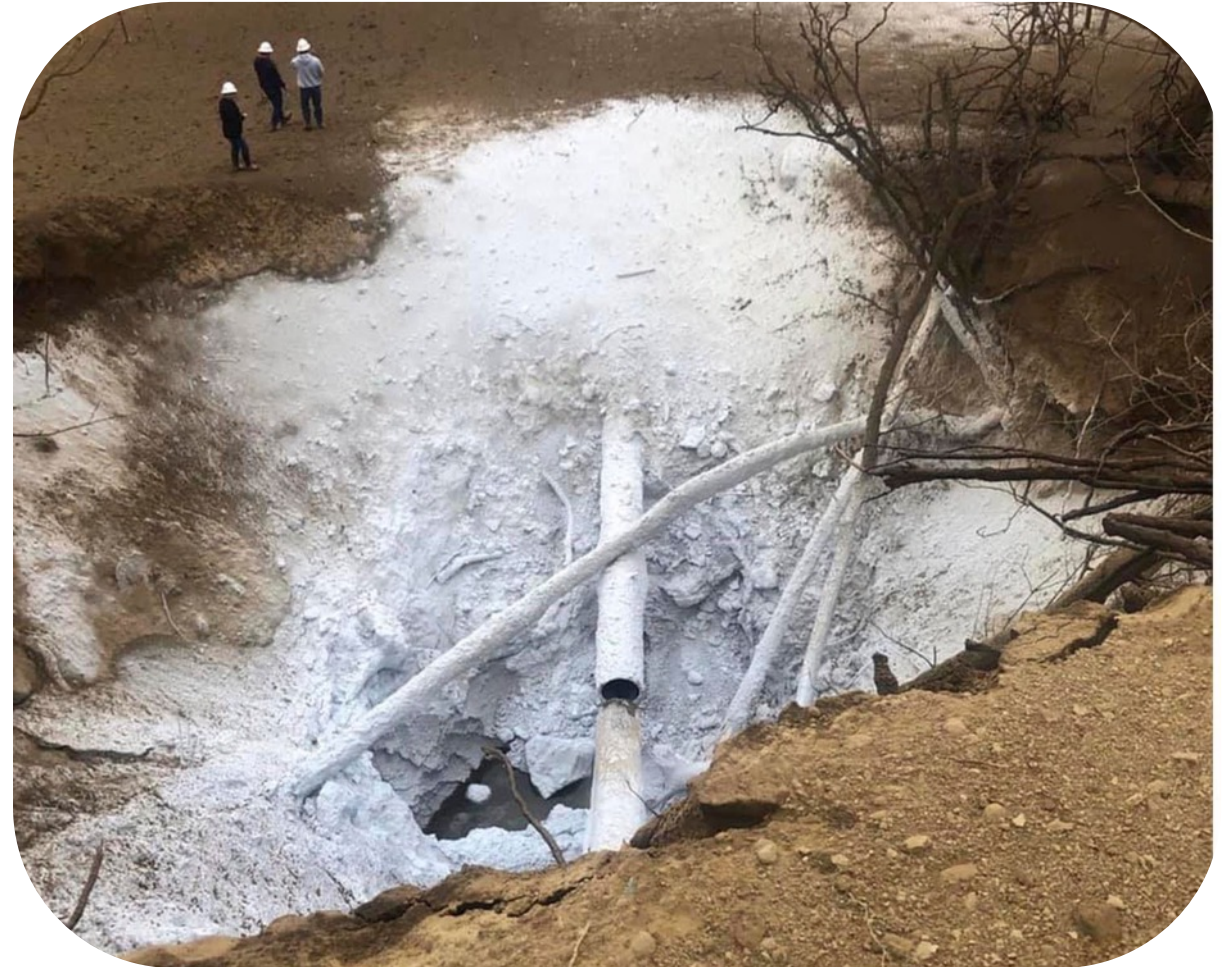
Denbury CO 2 pipeline rupture, Satartia, Mississippi, February 2020. Source: Huffington Post , April 2021.
