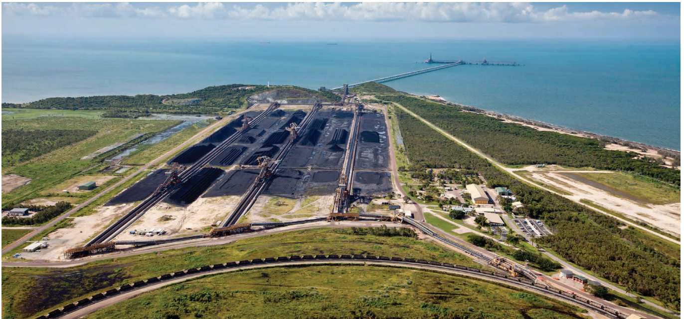
Figure 17: AAPCT – Coal Stockpile, Rail Link and Pier to T1
