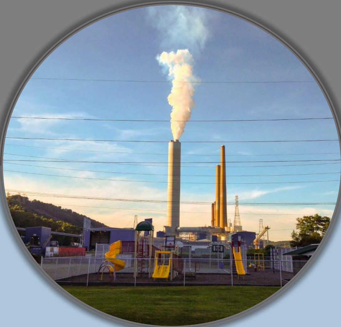
FirstEnergy's W. H. Sammis Plant, Stratton, OH
