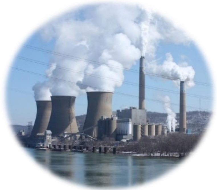
Bruce Mansfield Plant
