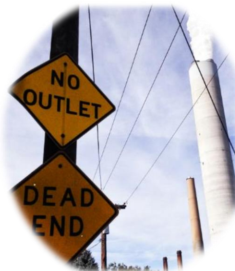
First Energy's Sammis plant
